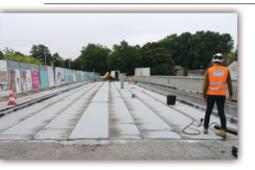
> Rincent Investigations has carried out tests by infrared thermography to check the waterproofing installation on a bridge.
